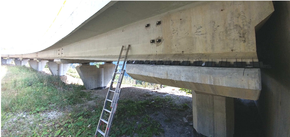
Figure 1. Test samples “Y” placed at bridge near Nová Bystrica – Vychylovka.
